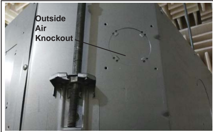
Figure 13. Typical Outside Air Knockout
